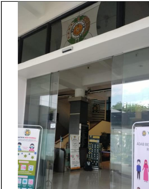
The Automatic Door Sensor System
